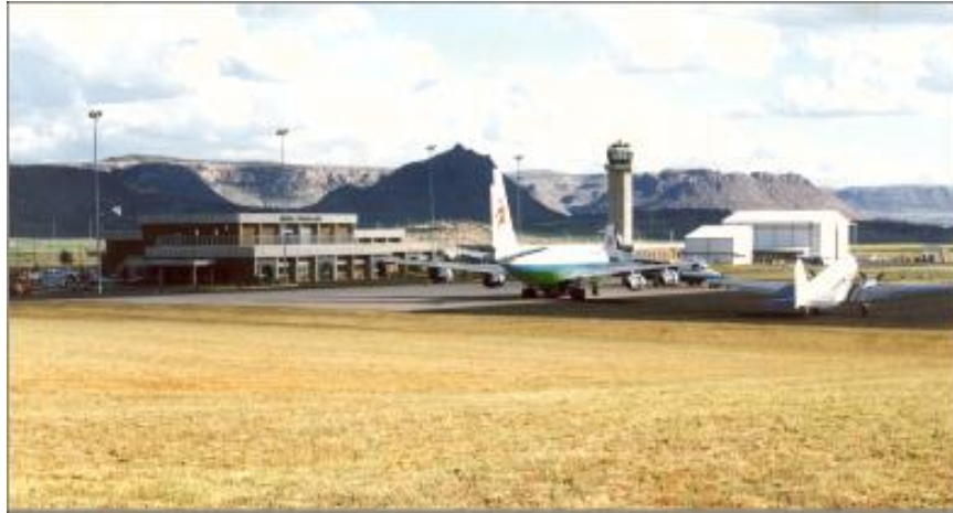
Figure 2: Panoramic view of the Moshoeshoe I International Airport Terminal Building
